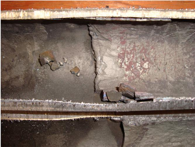
**FIGURE 2 – TYPICAL CORROSION OCCURRING DOWNSTREAM FROM FERRULE**
